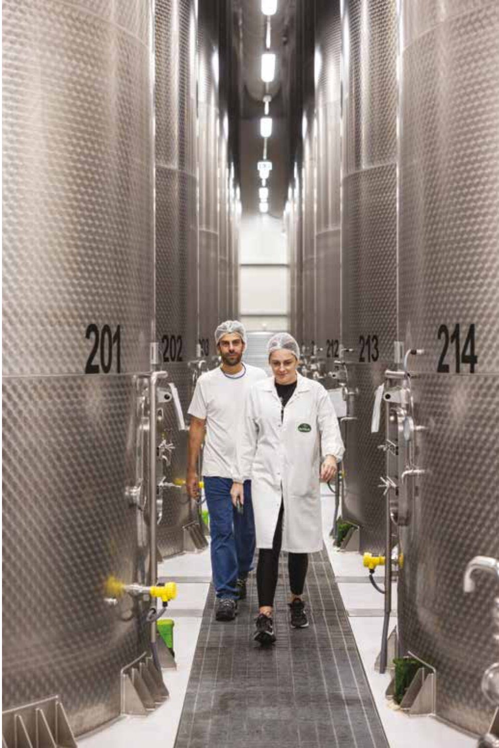
Warehouse B1: tanks in an air-conditioned environment
